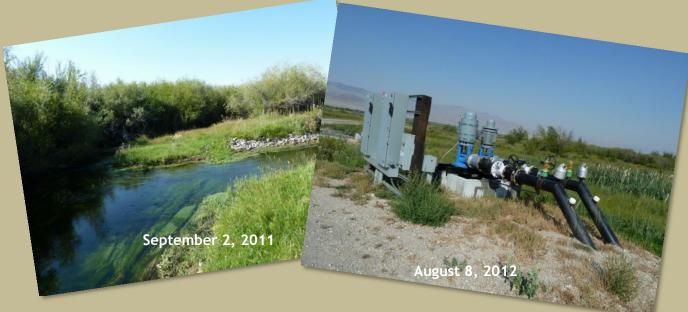
Patterson Big Springs Creek: Working with the Custer Soil and Water Conservation District, Idaho Fish and Game, the National Resource Conservation Service, and the water user, a diversion on Patterson Big Springs Creek was removed and a new pump was installed in a small non-fish bearing creek. A 20-year source switch agreement will protect 6 cfs in Patterson Big Springs Creek for high quality Chinook salmon spawning habitat.
