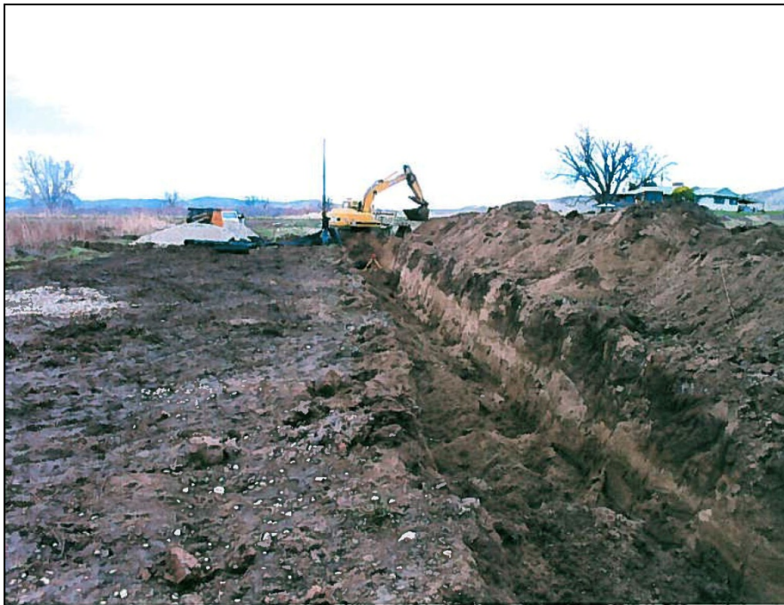
Photo: Canyon County Drainage District No. 2 replaced 1300 feet of failed drainage tile with a $35,000 loan provided by the Idaho Water Resource Board.
