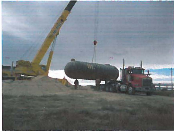
Removing one of the two 20,000 gallon storage tanks from the truck.
