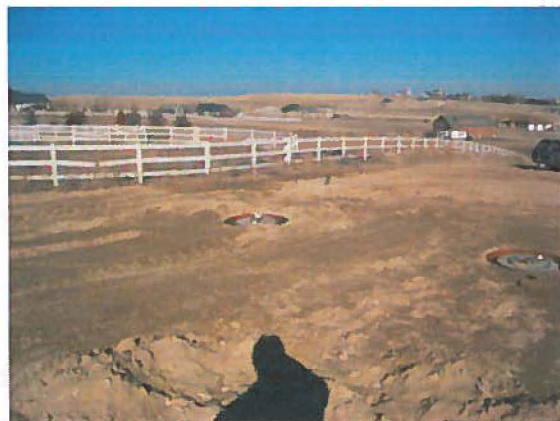
Both storage tanks installed and buried with only the access ports visible.
