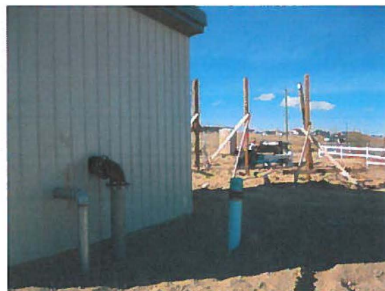
The piping coming from the pump house to the storage tanks.
