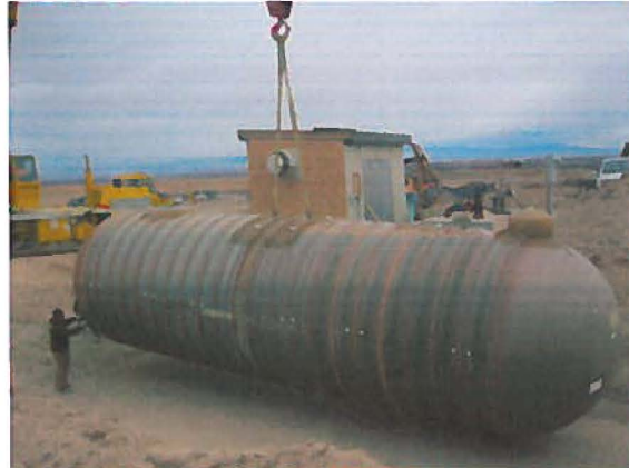
Placing the storage tank into the pre-dug pit.
