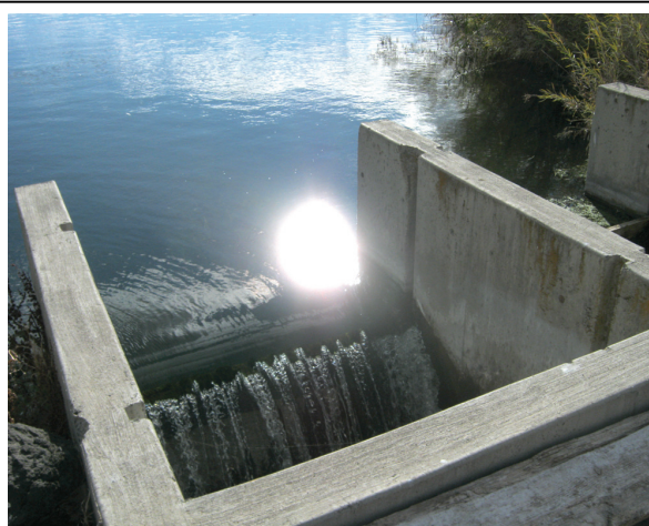
Headgate at Pristine Springs Hydropower Facility.
