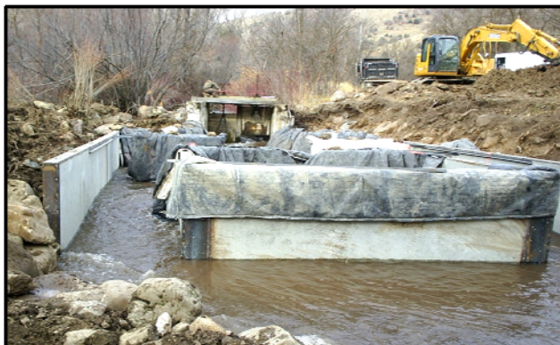
Preston Whitney Irrigation Company weir and headgate replacement, November 2009.
