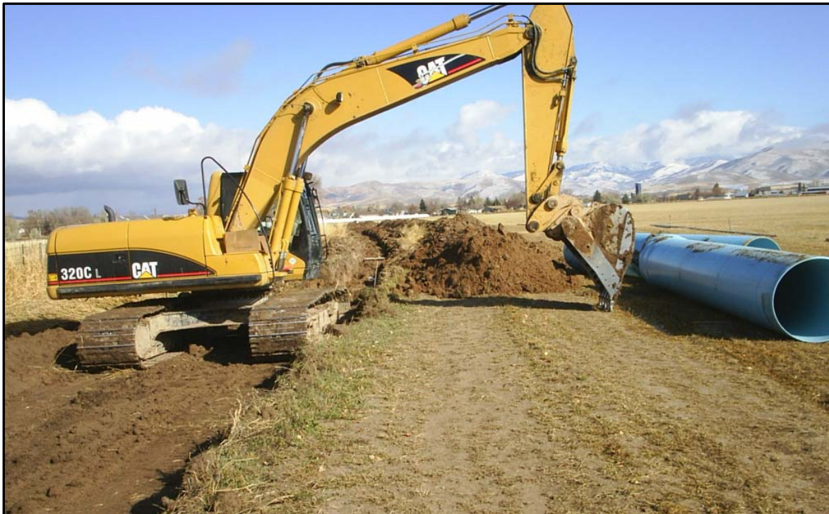
Construction on a new gravity pressurized mainline for Preston Whitney Irrigation Co. in Franklin County.
