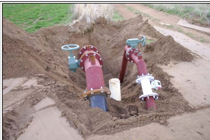
Preston Whitney Irrigation Company headgates and measurement devices for a new gravity pressurized pipeline.
