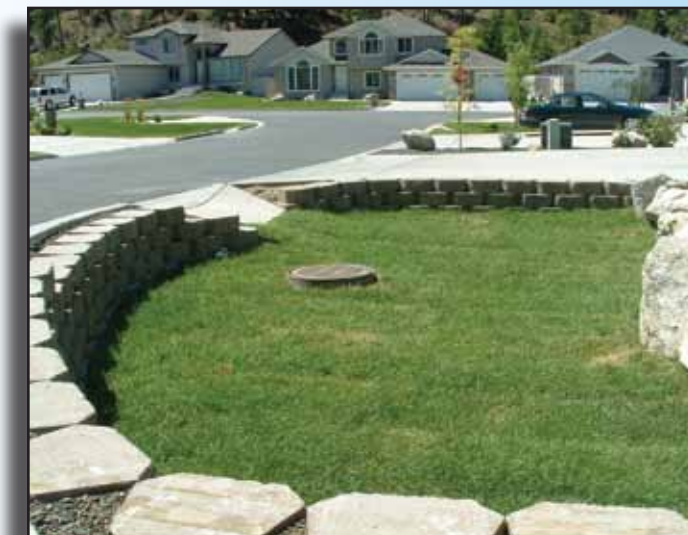
Stormwater swales and drywells recharge the Aquifer.
