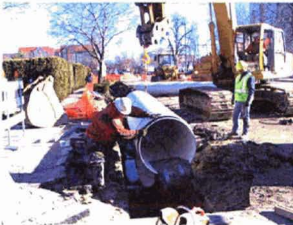
Above Left: Typical condition of the old covered canal sections. Above Right: Replacement covered canal sections being placed prior to the 2004 irrigation season. Below Right and Left: Rehabilitation of covered canal sections prior to the 2005 irrigation season. The space around the new pipe was filled with grout.
