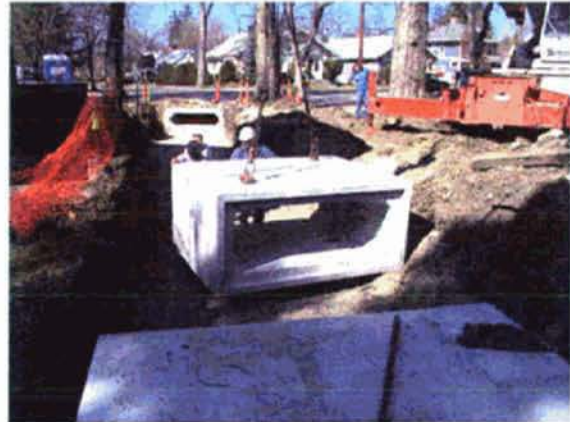
Above Left: Typical condition of the old covered canal sections. Above Right: Replacement covered canal sections being placed prior to the 2004 irrigation season. Below Right and Left: Rehabilitation of covered canal sections prior to the 2005 irrigation season. The space around the new pipe was filled with grout.
