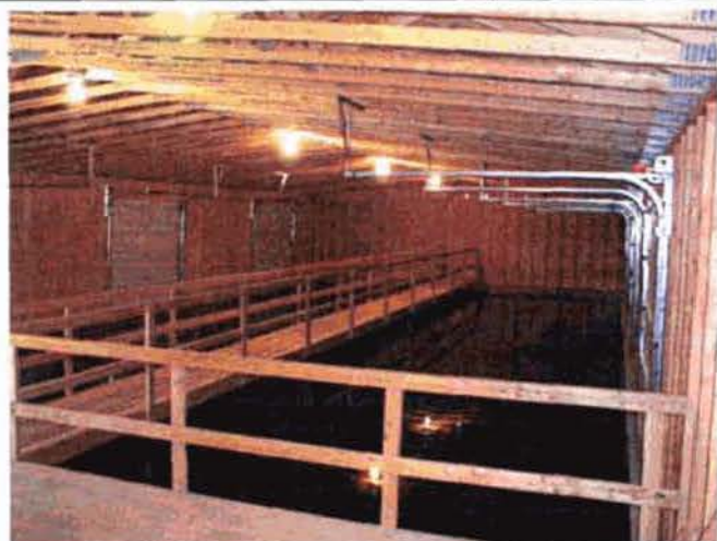
The Water Resource Board has assisted with the construction and improvement of several drinking water treatment plants around the state. This photograph shows the filter beds at the water treatment plant that serves the small town of Naples. This plant treats water from 20-Mile Creek to drinking water standards prior to delivery for use.
