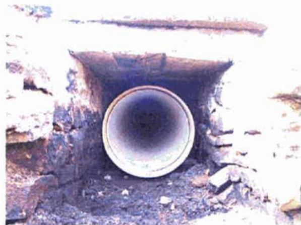
Above Left: Typical condition of the old covered canal sections. Above Right: Replacement covered canal sections being placed prior to the 2004 irrigation season. Below Right and Left: Rehabilitation of covered canal sections prior to the 2005 irrigation season. The space around the new pipe was filled with grout.
