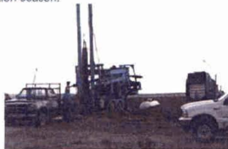
Above: Deepening of one the Jefferson Irrigation Company's ground water wells. Below: Deepened well in use.
