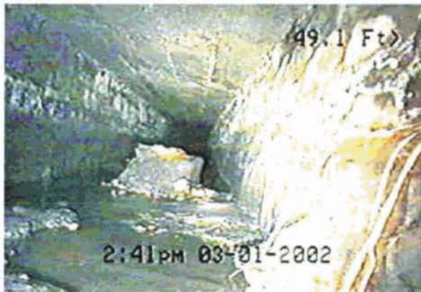
Above Left: Typical condition of the old covered canal sections. Above Right: Replacement covered canal sections being placed prior to the 2004 irrigation season. Below Right and Left: Rehabilitation of covered canal sections prior to the 2005 irrigation season. The space around the new pipe was filled with grout.
