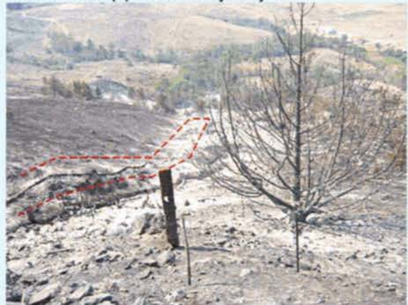
Above: Spring collection box severely damaged by fire. Below: Water pipeline destroyed by fire.
