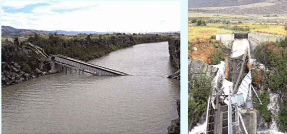
Above: Two views of the collapsed Last Chance Canal Company flume.
