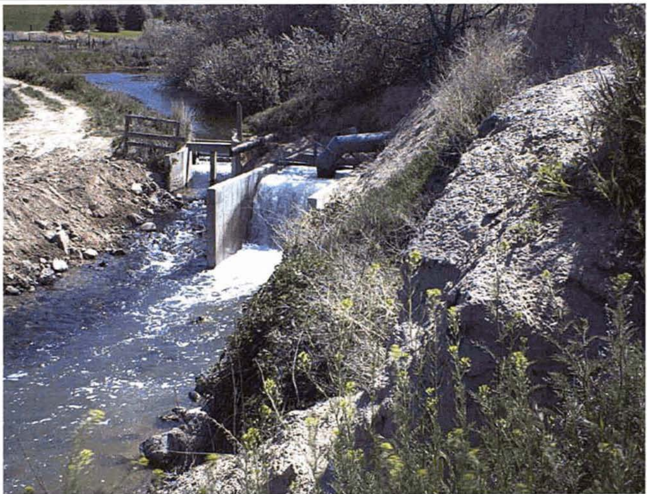
Photograph showing the North Snake Groundwater District’s “Sandy Pipeline” delivering rented surface water to the Curren Ditch, one the major spring-fed canals in the Hagerman area. The Idaho Water Resource Board provided financing for this project. Additional mitigation and water management projects will be necessary to help solve the Eastern Snake Plain Aquifer situation.
