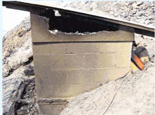
Above: Spring collection box severely damaged by fire. Below: Water pipeline destroyed by fire.
