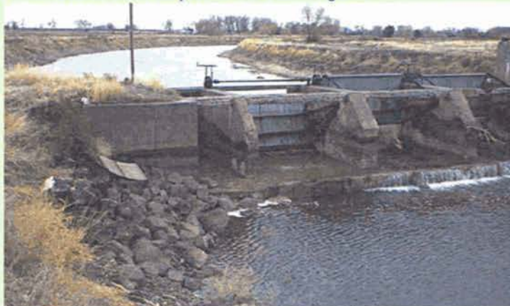
Above: Condition of the diversion structure prior to reconstruction. Below: Construction of the new structure underway by Cannon Construction (Blackfoot).
