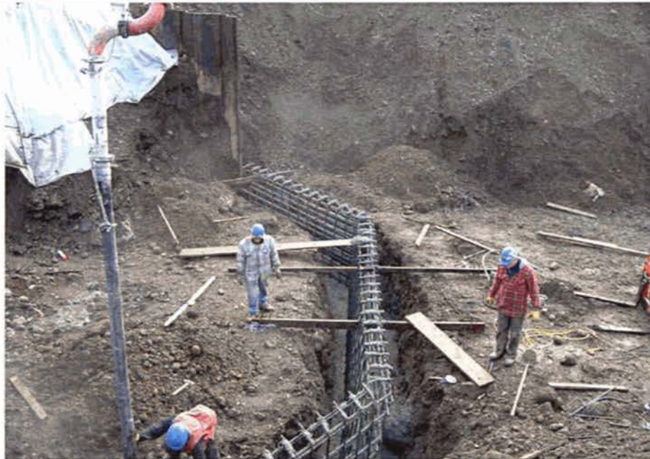
Cut-off wall being constructed during the replacement of the Twin Lakes Dam. The work is scheduled to be complete by spring of 2005. The dam, originally constructed in 1906, is owned by the Twin Lakes-Rathdrum Creek Flood Control District and provides for the storage of 9,090 acre-feet of water. The Idaho Water Resource Board is providing financing for the project, which will be repaid over a 15-year term by a property tax assessment on all properties within the District.
