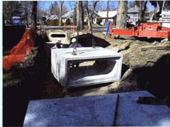
Above Left: Typical condition of the old covered canal sections. Above Right: Replacement covered canal sections being placed prior to the 2004 irrigation season. Additional sections of the canal will be replaced or rehabilitated prior to the 2005 irrigation season.
