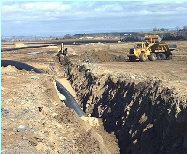
Above Left: Installation of 36" HDPE pipe during construction of the pipeline. Above Right: the completed pipeline delivering 32 cfs into the Curren Ditch in the Hagerman Valley, which is fed by the Curren Tunnel Spring. Below: Project location map.
