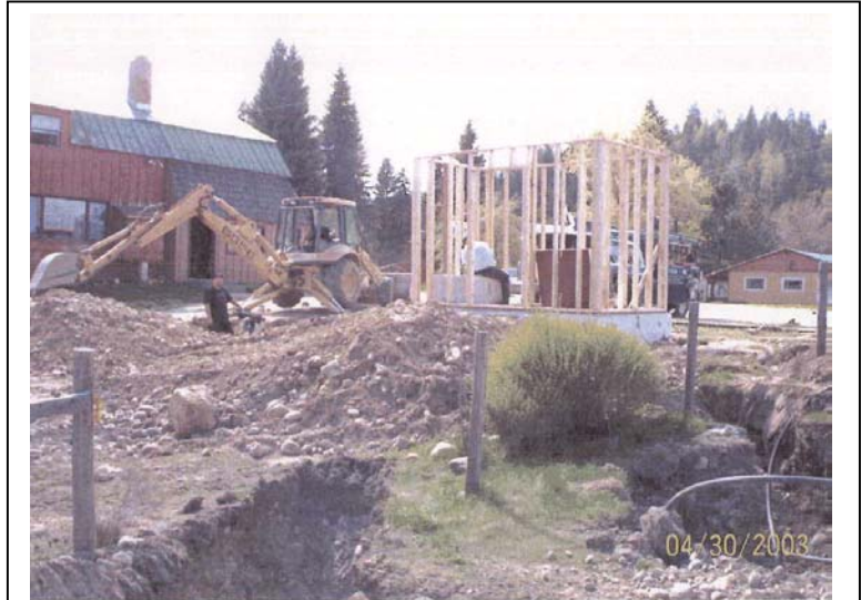
New pump house and water lines under construction for the Deep Creek Water Association. This system delivers water to the small community of Deep Creek. The project consisted of improvements mandated by the Department of Environmental Quality. The contractor was Deal Pump & Electric (Sandpoint). The Water Resource Board's project loan will be repaid by the Association over 10 years.
