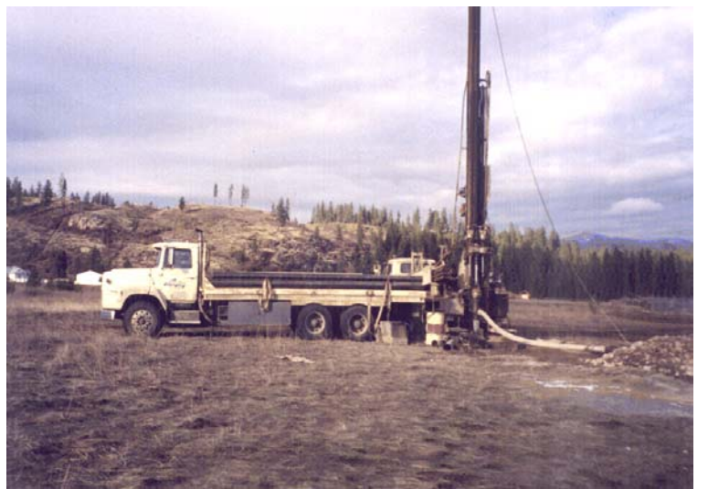
New well being drilled for the Hoyt Bluff Water Association by United Well Drilling (Hayden). The Association delivers domestic water to 70 homes near Rathdrum. The construction loan will be repaid by the Association over a 15-year term.
