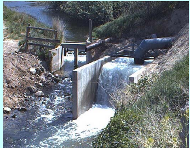
Above Left: Installation of 36" HDPE pipe during construction of the pipeline. Above Right: the completed pipeline delivering 32 cfs into the Curren Ditch in the Hagerman Valley, which is fed by the Curren Tunnel Spring. Below: Project location map.
