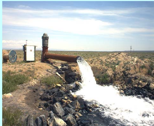
Above Left: Construction of the replacement Well No. 1. Above Right: The deepened Well No. 12 pumping water into the irrigation canal for delivery to the farm lands. Below: Project location map.
