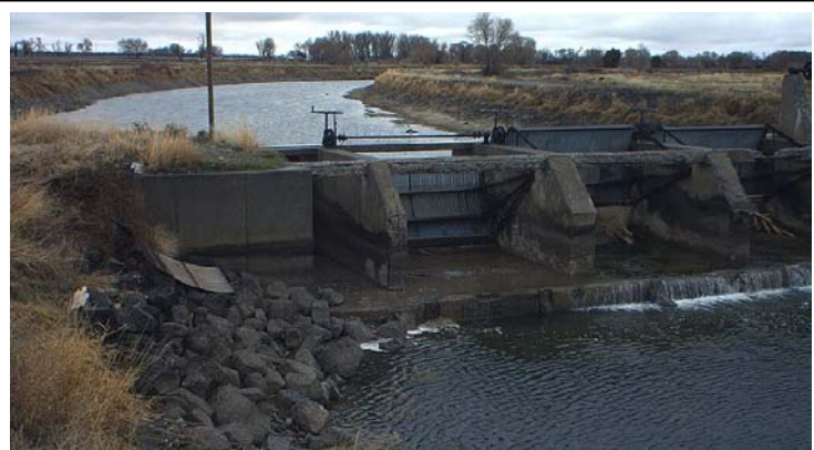
Diversion structure on the Aberdeen-Springfield Canal Company's Feeder Canal that diverts flows into the Main Canal. The Water Resource Board has agreed to finance the replacement of this critical, severely deteriorated structure that has been in use since the 1930's. In the event of failure of this structure, water could not be delivered to 60,000 acres of highly productive farmland, causing severe economic impacts to southeastern Idaho.
