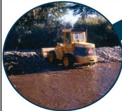
1994 Common practice of building a gravel diversion dam to redirect river flow down a ditch to irrigate hay fields. This occurred multiple times each irrigation season due to changing river flows that would deconstruct the dam.
