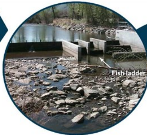
1998 Post-construction of new concrete weir at L6 diversion eliminating the need for machinery to construct the gravel dam. Dam includes a fish ladder bay but water rights continued to dewater the river at low flow periods.
