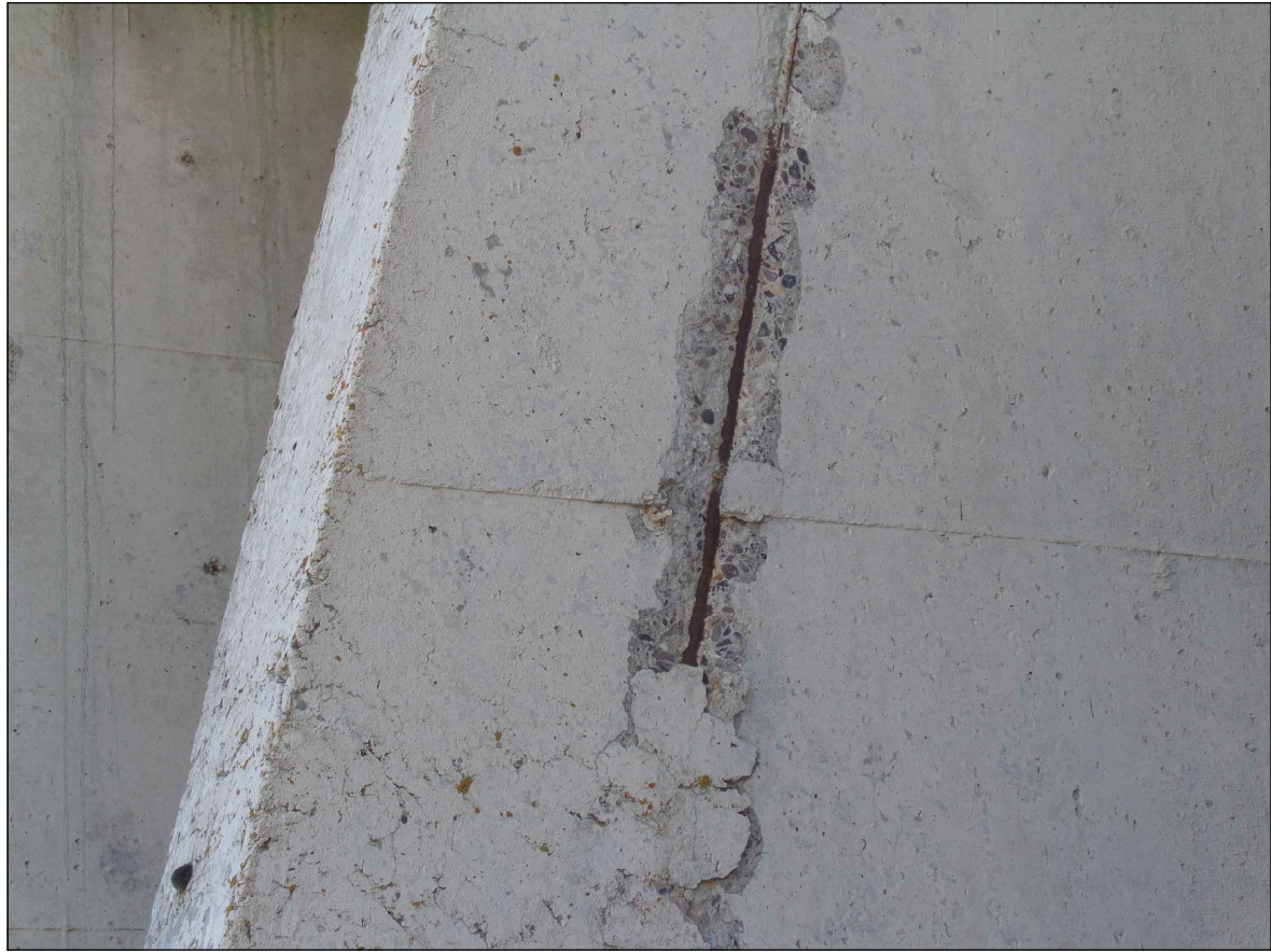
TYPICAL VIEW OF REBAR TO BE COATED PER SPECIAL PROVISION S501-30A
