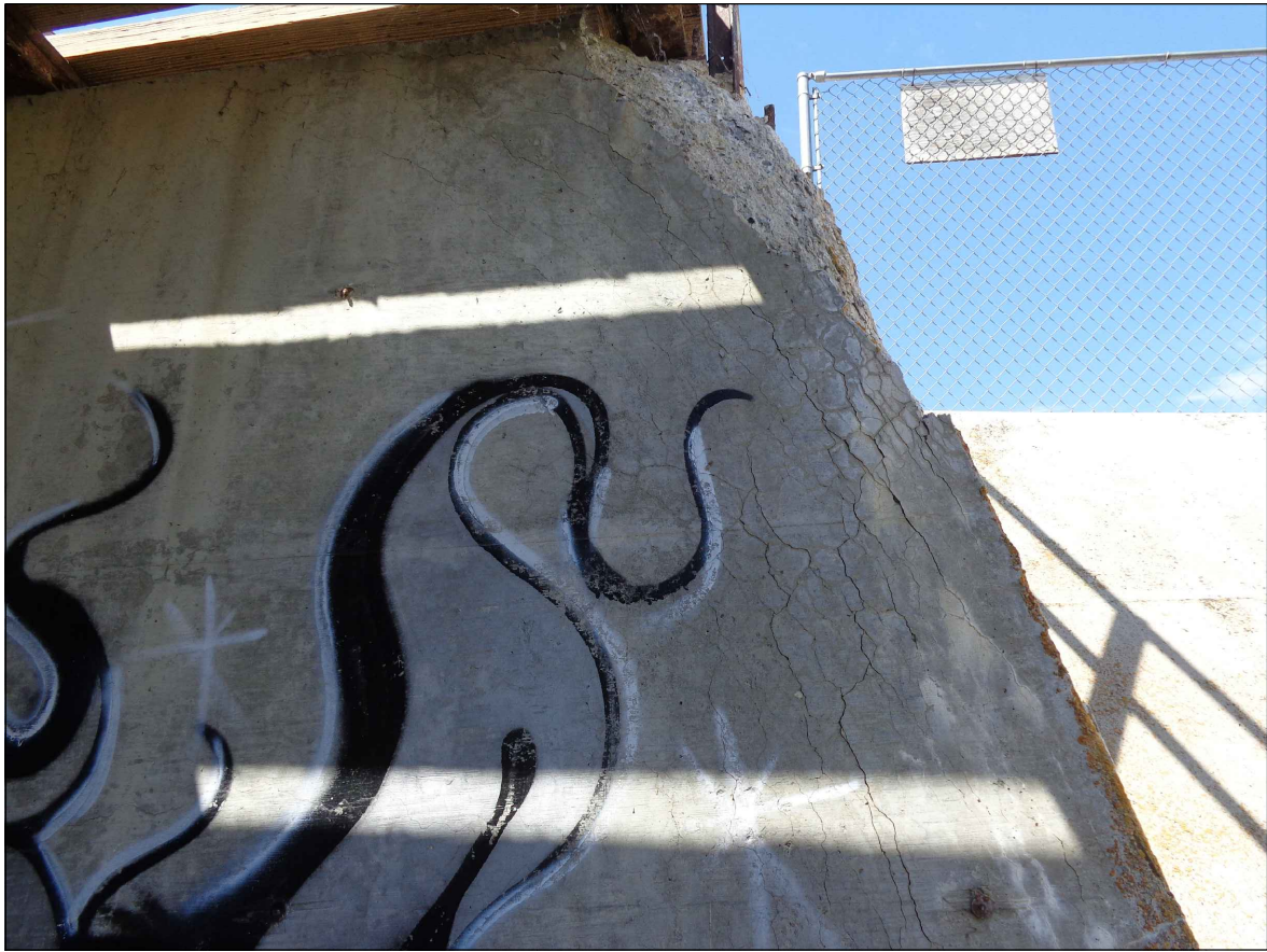
TYPICAL VIEW OF CONCRETE SURFACE TO BE REPAIRED PER SPECIAL PROVISION S501-51A
