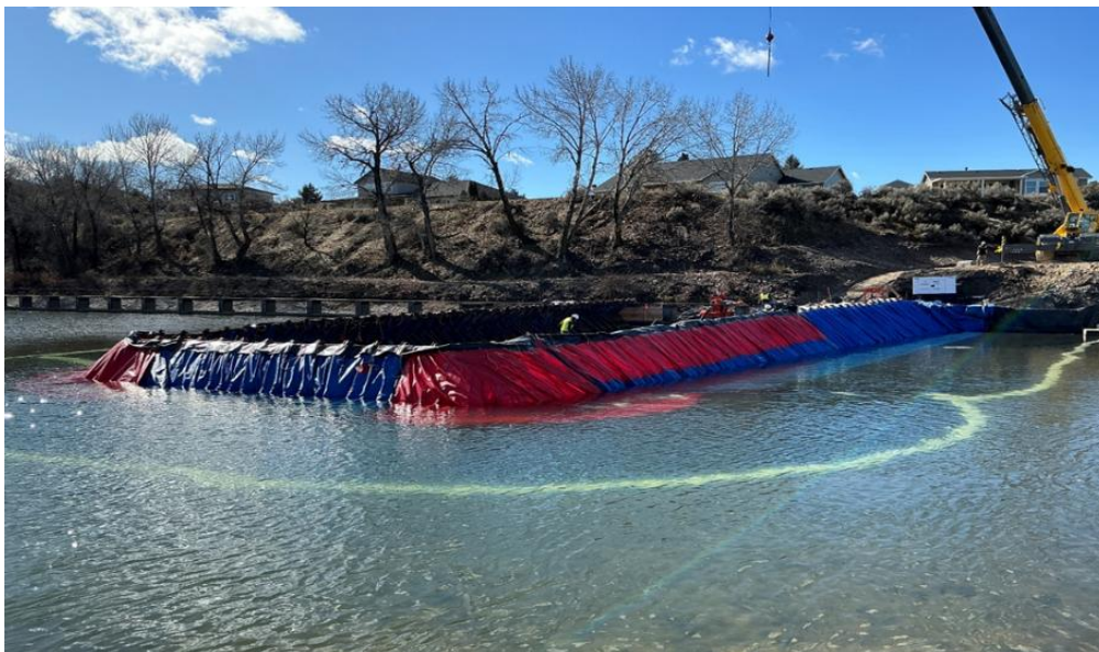
Figure 7 PortaDam installed across half of the Boise River in February 2025
