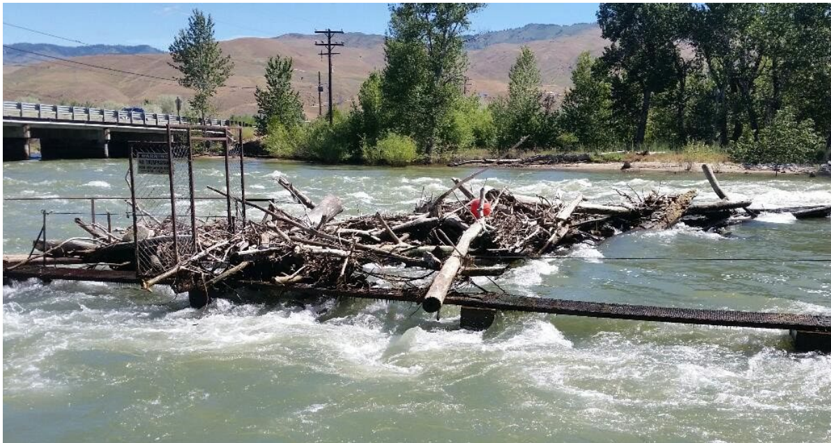
Figure 10 Photo taken on June 18, 2017. The Diversion structure has collected debris, which cannot be removed safely during flood conditions.
