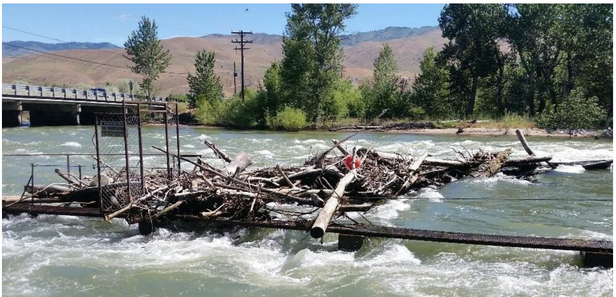
Figure 3 Photo taken on June 18, 2017. The Diversion structure has collected debris, which cannot be safely removed during flood conditions. The flood risk reduction benefits are the project are detailed in this proposal.
