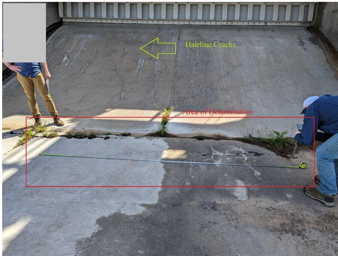
Figure 9: Service Spillway at Milner Dam Area of Delamination and Hairline Cracks.
