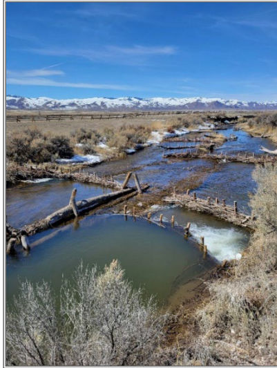
The images on the left were taken in March 2023 during an Idaho Fish and Game sponsored tour of proposed and current stream channel restoration work in the Upper Pahsimeroi River basin. The image on the far-left shows stream bank erosion that can lead to significant property loss without proper stream restoration work. The image on the right is of recently constructed beaver dam analogs which help reduce erosion from high flows and improve bank stability by promoting riparian growth. Photos courtesy of John Loffredo, IDWR.
