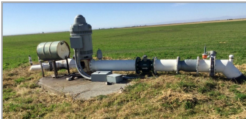
A groundwater irrigation well with an installed flow meter located on the Eastern Snake River plain. Image courtesy of the Water Distribution Section.
