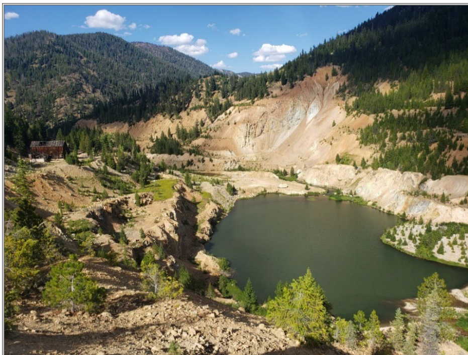
Stibnite Mine in Valley County. Stibnite’s mine tailings impoundment structure is included in the nearly 20 impoundment structures inspected by IDWR Dam Safety staff. Photo courtesy of Angie Hansen, IDWR.
