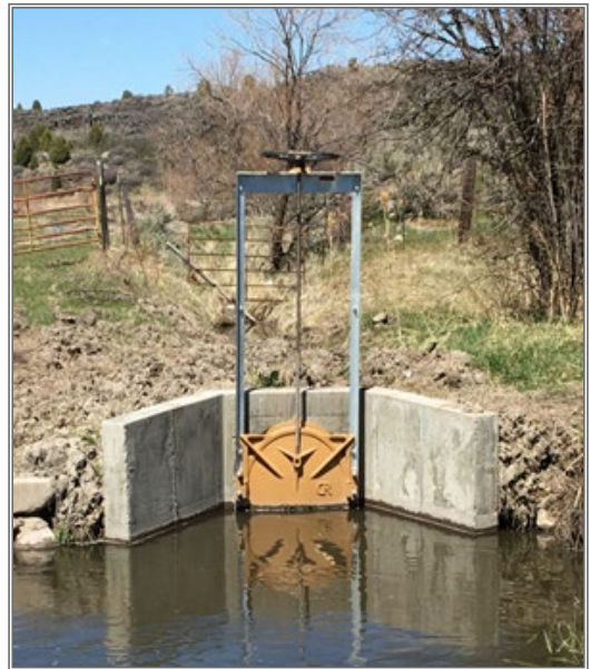
A recently installed headgate used by a watermaster to control a diversion on the Portneuf River. Image courtesy of the Water District Program.
