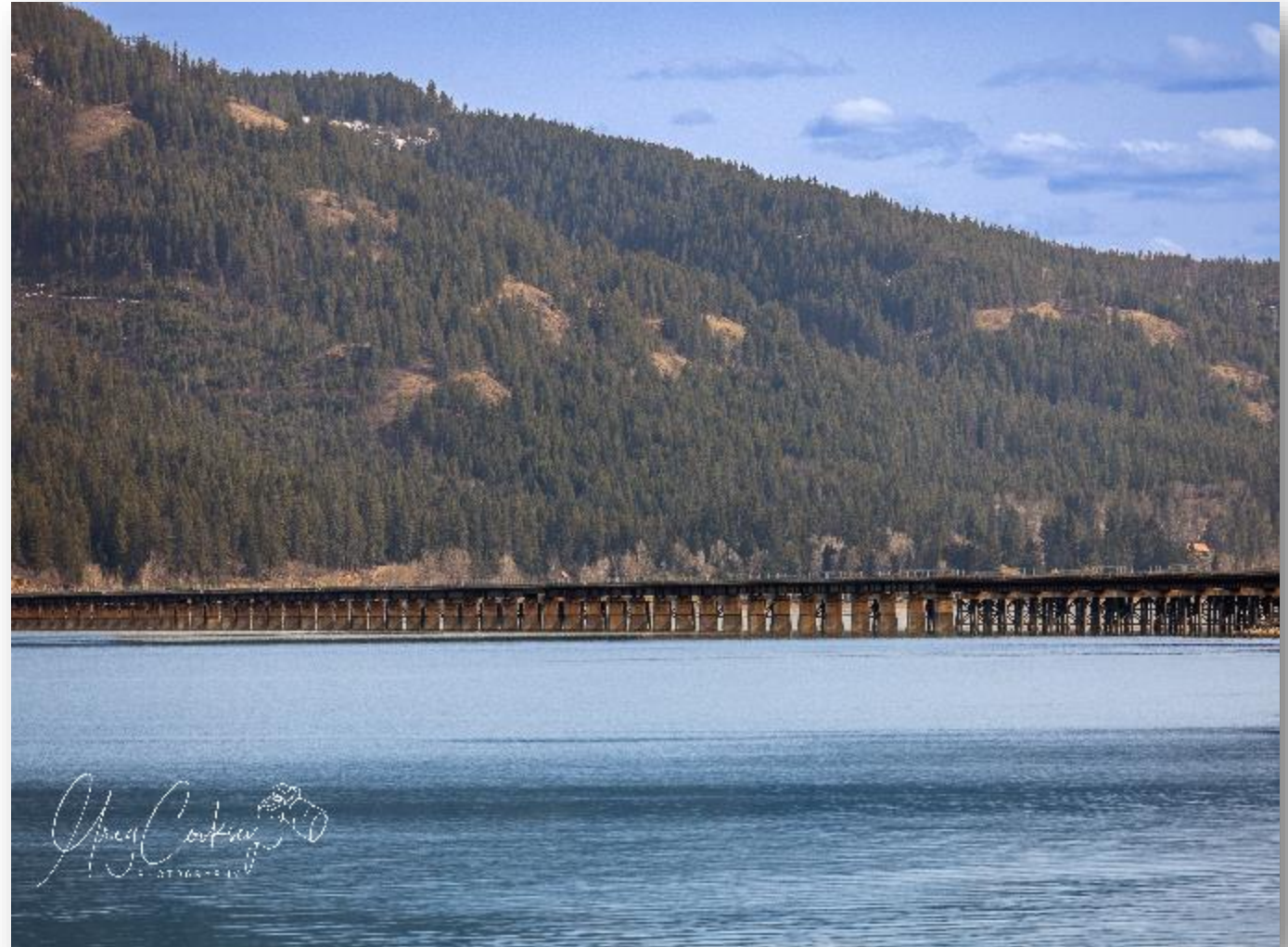
Trestle by Long Bridge in Sandpoint Photo courtesy of Greg Cooksey, Northern Region
