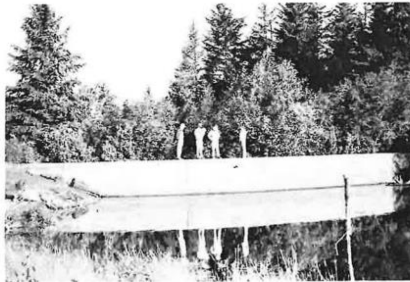
Photograph No. 2 - Upstream face of dam. August 3, 1978.
