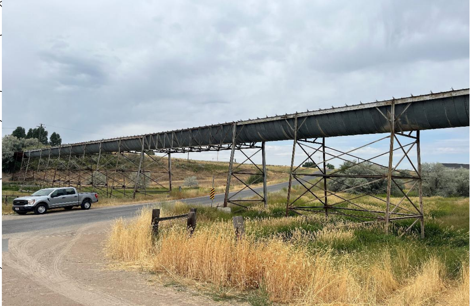
Flume near Preston
