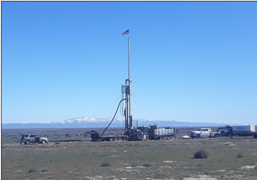
Figure 6: MH 2 being drilled by Cold Steel Drilling in March 2024.
