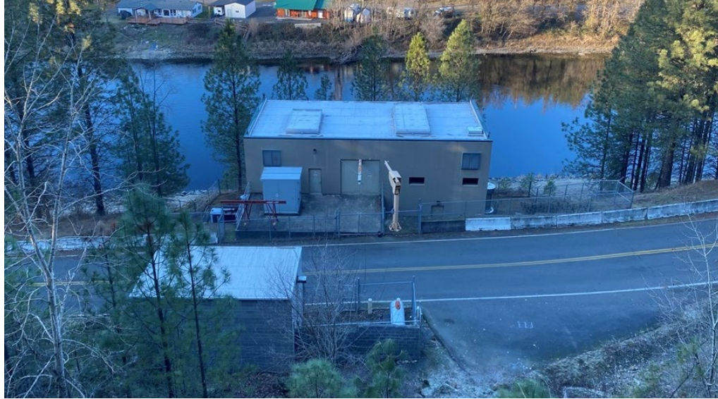
Figure 1: Dworshak Small Hydro Plant
