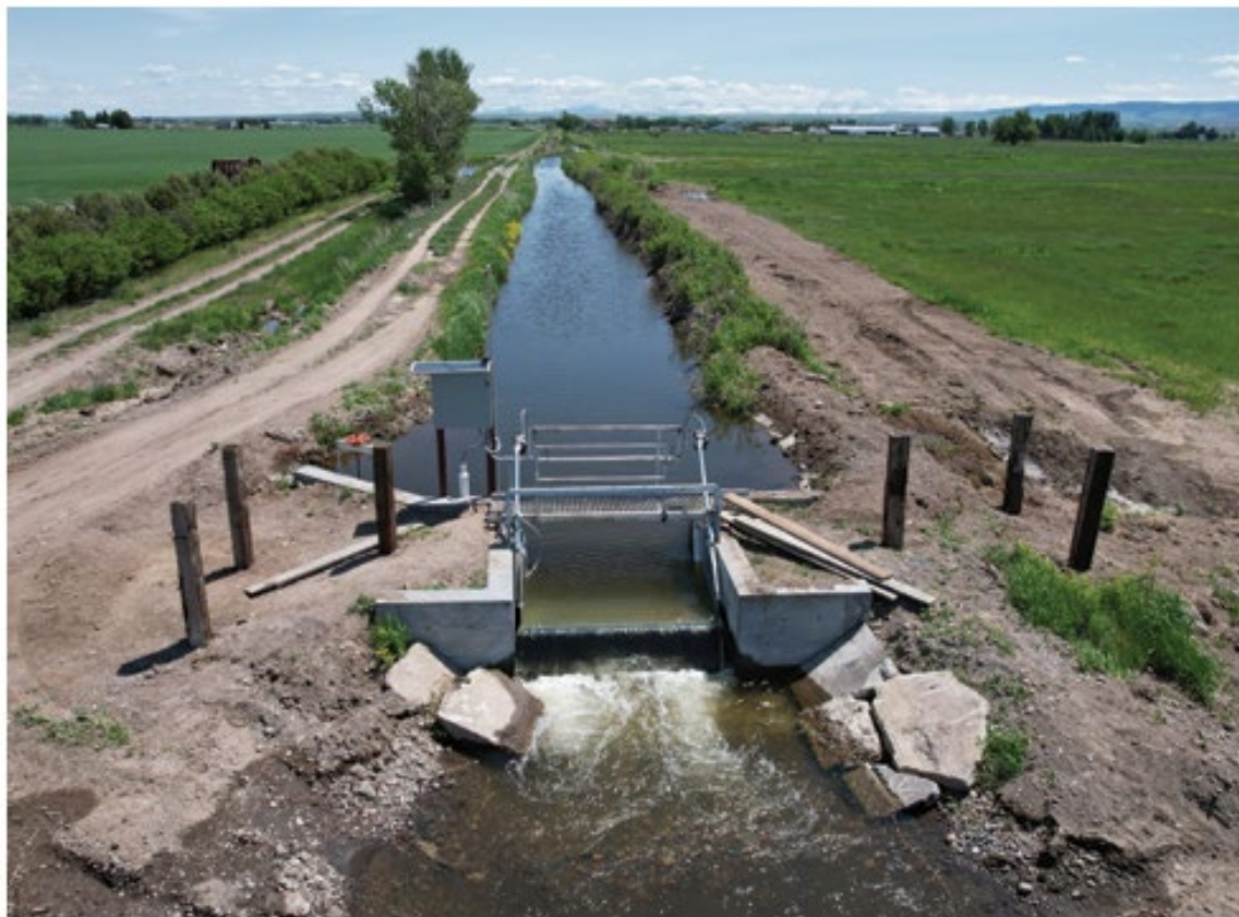
New concrete structure and canal automation equipment installed on the Middle Branch of the Fall River canal system. (Photo courtesy Aaron Dalling, FMID)
