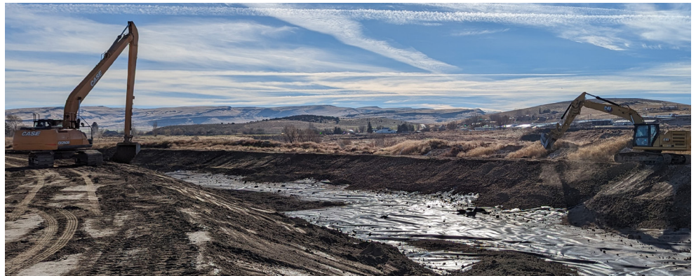
Above, location of canal-lining project near Rock Creek gravel pits. Below, contractors prepare the canal embankments for the geomembrane liners. (TFCC photos)
