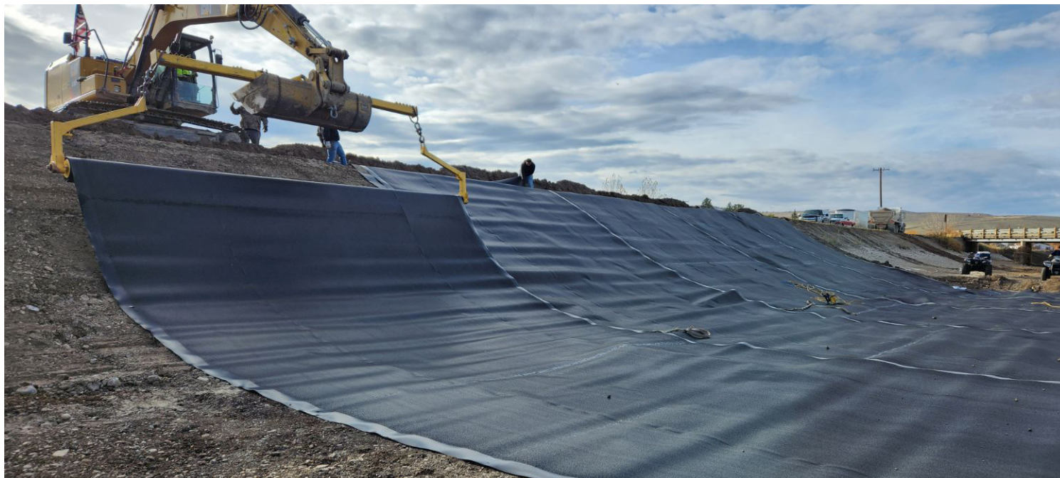
Contractors unfurl large sheets of geomembrane canal liner on the 105-foot-wide High Line Canal. (courtesy TFCC)
