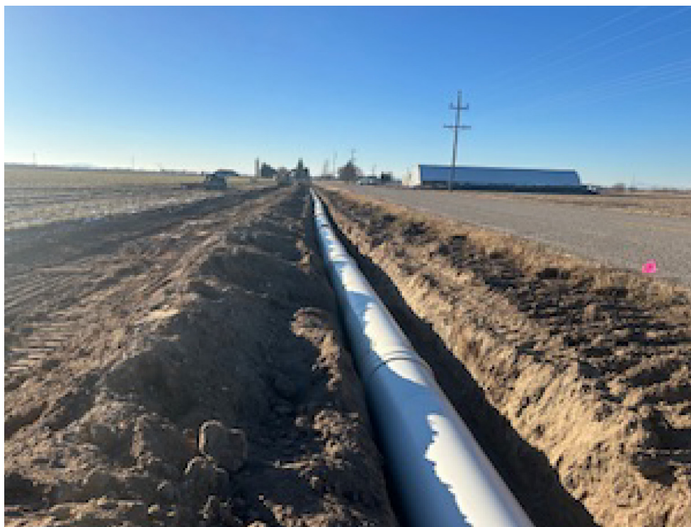
New irrigation pipeline for Teton Irrigation Canal Co. is ready for the 2025 irrigation season (photo courtesy Dan Nedrow).
