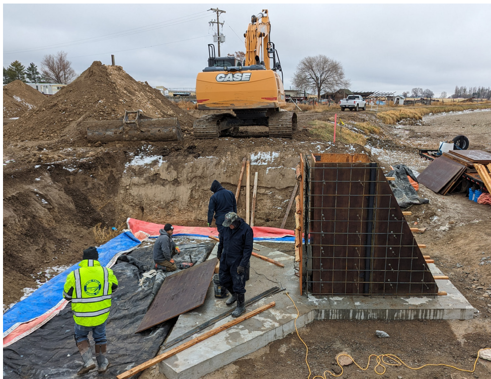
Contractors pour concrete for Rubicon water measurement device in the Clover Tract served by the Twin Falls Canal Co., southwest of Filer. (photo courtesy Twin Falls CC).
