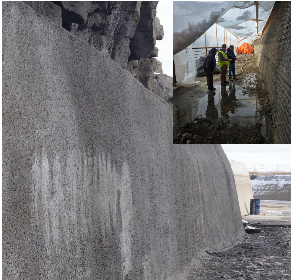
Recently completed canal walls are sealed with shotcrete and ready for efficient irrigation use in the spring of 2026. Inset photo: Heated tent structure, kept at a temperature of 60 degrees, allows the shotcrete walls to cure for four days following the application. (Photo by Steve Stuebner/IWRB)
