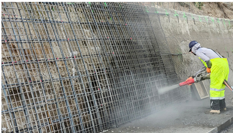
Construction specialist applies shotcrete, a mix of cement, sand, and aggregate mix pneumatically projected through a hose at high velocity onto the walls of the North Side main canal below Milner Dam. (Photo courtesy North Side Canal Co.)
