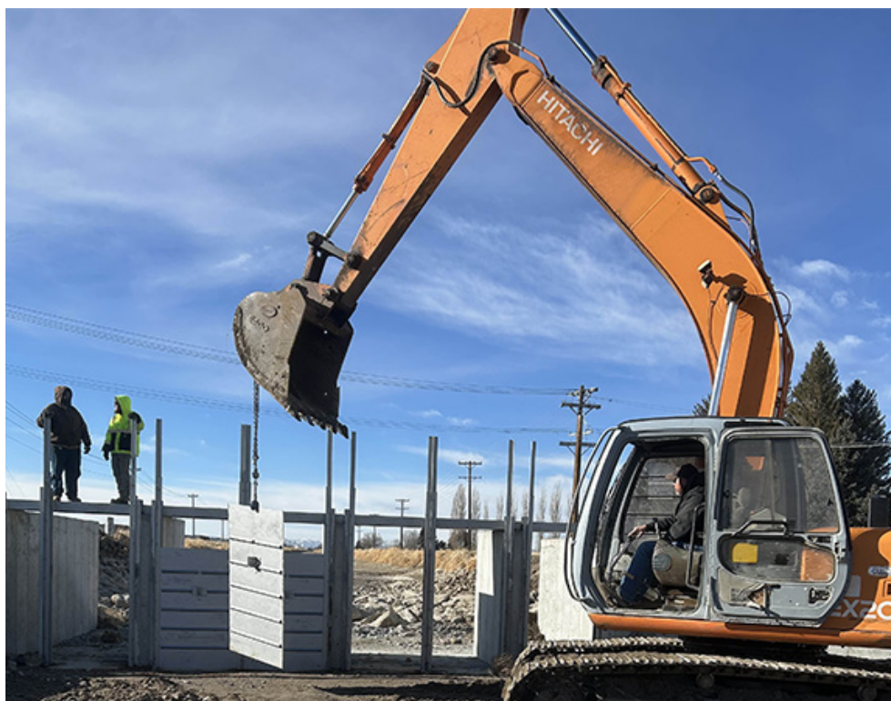
Construction crew installs the gates on a new check/diversion structure in the winter of 2024-25 for Minidoka Irrigation District. (photo courtesy MID).
