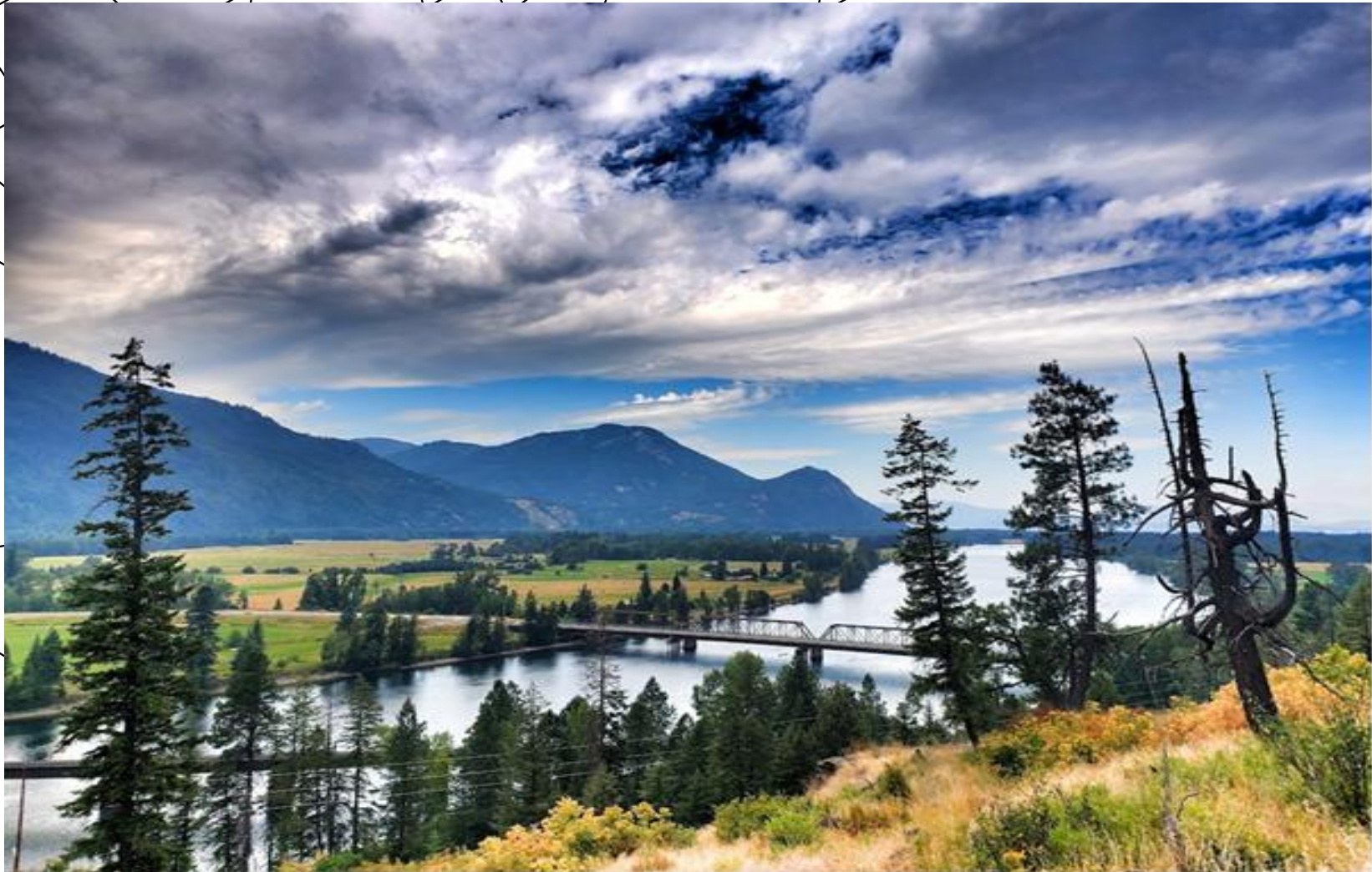
Clark Fork River Bridge
