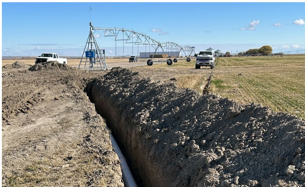
New pipeline in place replaces the old lateral ditch, connecting directly to a pivot in a farm field, eliminating seepage losses. (Photo courtesy Jefferson Irrigation Co.)
