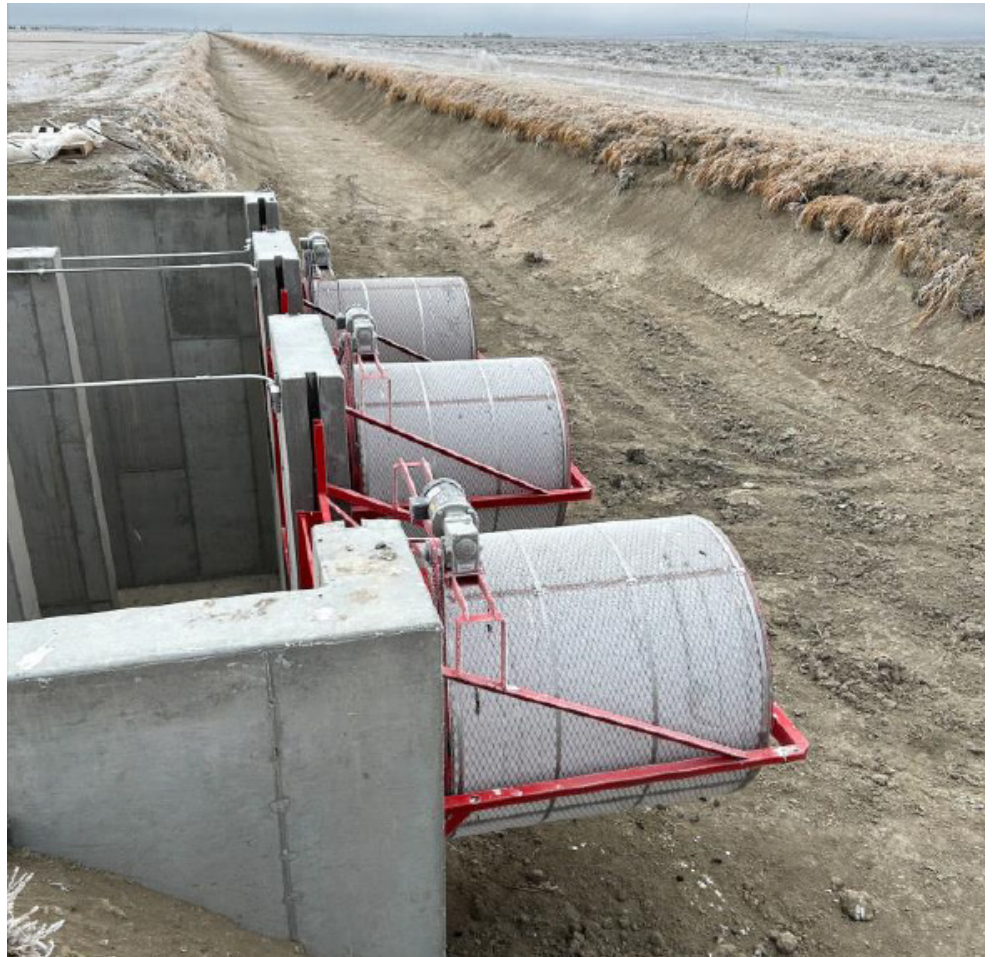
New concrete pumping station structure and intake screens are in place during construction in the winter of 2024-25. (Courtesy Jefferson Irrigation Co.)
