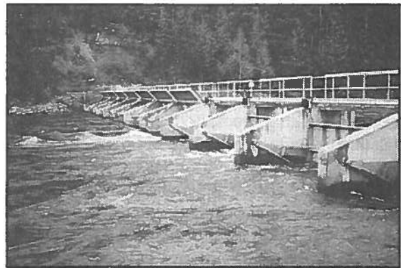
Figure 7. Priest Lake Outlet Structure
