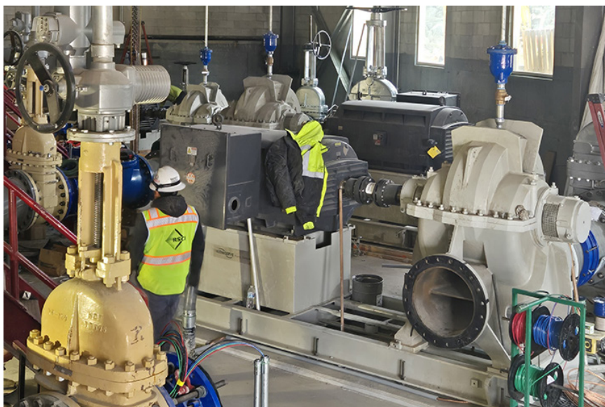
New pumps getting installed inside the Falls Irrigation District pumphouse adjacent to American Falls Dam. (photo courtesy Shawn Tischendorf)
