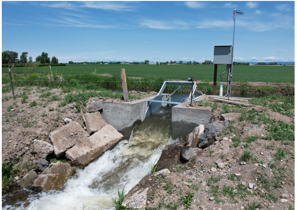
New concrete structure and canal automation equipment installed on the Middle Branch of the Fall River canal system allowed the canal co. to eliminate a section of redundant canal, saving water and improving efficiency. (Photo courtesy Aaron Dalling, FMID)
