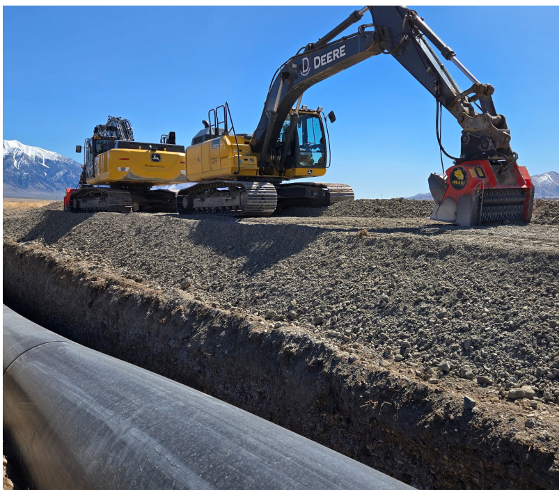
New HDPE pipeline installed in the Burnett Canal by contractors for the Big Lost Irrigation District. (photo courtesy Moj Broadie)
