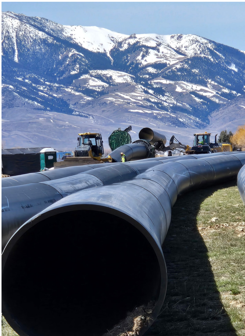
HDPE pipeline staged and ready for placement in the Burnett Canal. (Courtesy BLRID)
