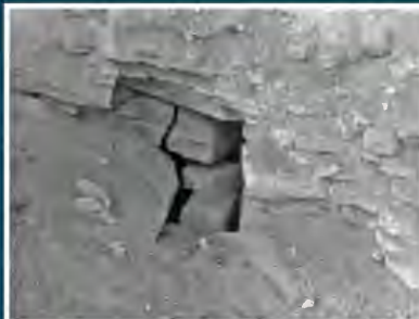
PS49-187-5201 NA Teton Dam, Teton Project, Idaho A void in the right abutment to be grouted at elevation 5140, 250 feet upstream, station 15+30. Morrison-Knudsen Company, Inc. and Peter Kiewit Sons' Company, Specifications No. DC-6910. 11/15/74 Bureau of Reclamation photo by B. Bockstruck
