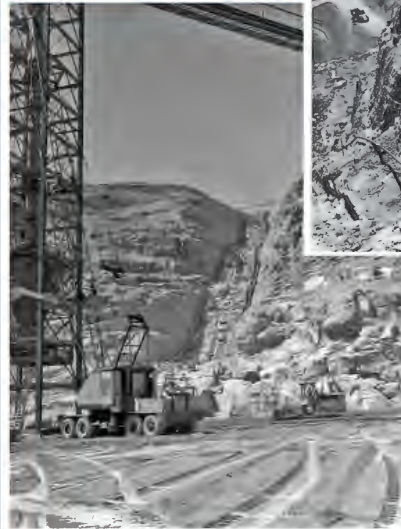
P549-147-4886 NA Teton Dam, Teton Project, Idaho Right abutment keyway showing drill track on the grout cap and access stairway on the upstream side. Morrison-Knudsen Company, Inc. and Peter Kiewit Sons' Company, Specifications DC-6910. 8/26/74 Bureau of Reclamation photo by B. Bockstruck
