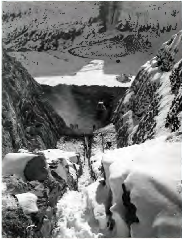
P549-147-4886 NA Teton Dam, Teton Project, Idaho Right abutment keyway showing drill track on the grout cap and access stairway on the upstream side. Morrison-Knudsen Company, Inc. and Peter Kiewit Sons' Company, Specifications DC-6910. 8/26/74 Bureau of Reclamation photo by B. Bockstruck
