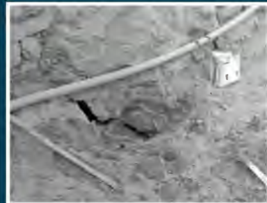
PS49-147-5216 NA Teton Dam, Teton Project, Idaho View of open joint on the right abutment at elevation 5142, station 14+52, 90 feet upstream ready to be grouted. Morrison-Knudsen Company, Inc. and Peter Kiewit Sons' Company, Specifications No. DC-6910. 11/14/74 Bureau of Reclamation photo by B. Bockstruck
