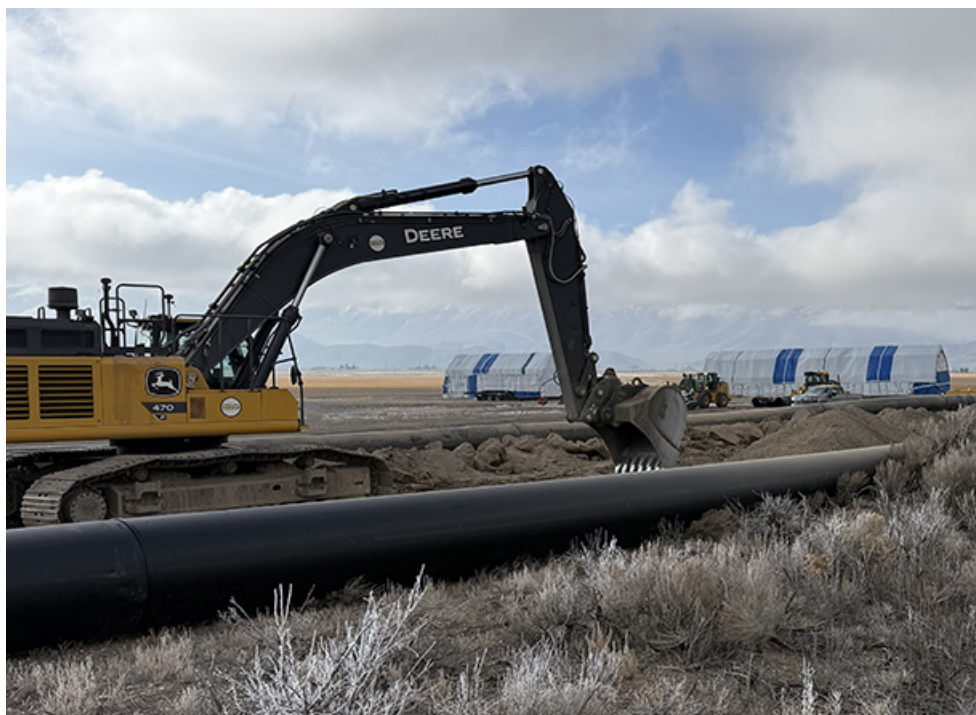
Construction crew installs HDPE pipeline in the Blaine County Canal Co. irrigation system near Howe during the winter of 2025-26 (photo courtesy Rory Pancheri).
