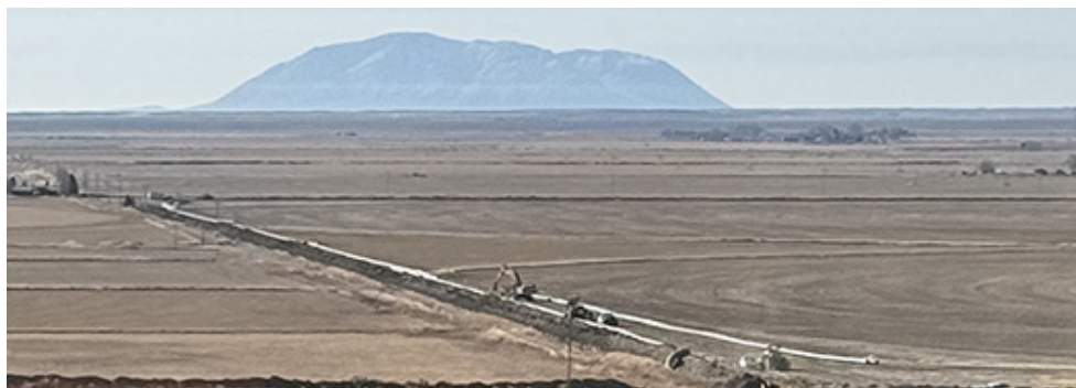
Above, HDPE pipeline in place in a deep trench after each section of pipe has been heat-sealed together. Below, a broader view of the project installation with Big Southern Butte in the background. (Photos courtesy Rory Pancheri, BCCC)
