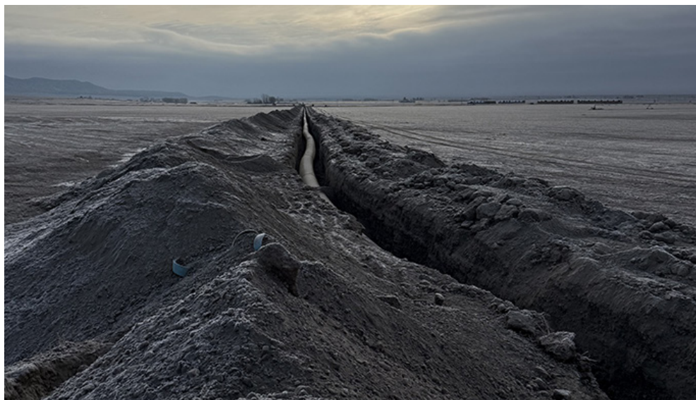
Above, HDPE pipeline in place in a deep trench after each section of pipe has been heat-sealed together. Below, a broader view of the project installation with Big Southern Butte in the background. (Photos courtesy Rory Pancheri, BCCC)
