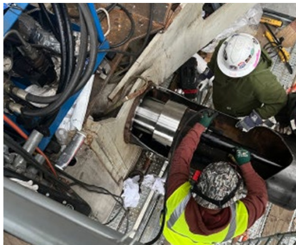
Above left, new trunnion pin ready for installation. Right, workers install a pin and bushing assembly on a spillway gate. (photos courtesy Bureau of Reclamation)
