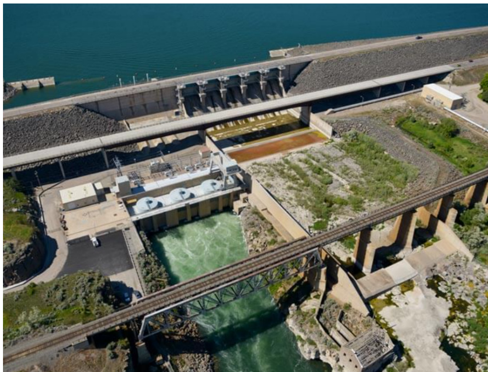
Overhead view of American Falls Dam, spillway and powerhouse. (Courtesy Idaho Power Co.)
