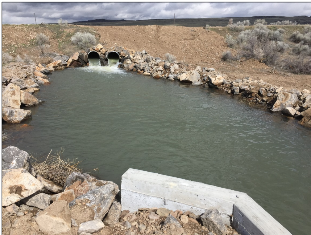
Figure 4. Stilling pool upstream of weir at BLM Pit
